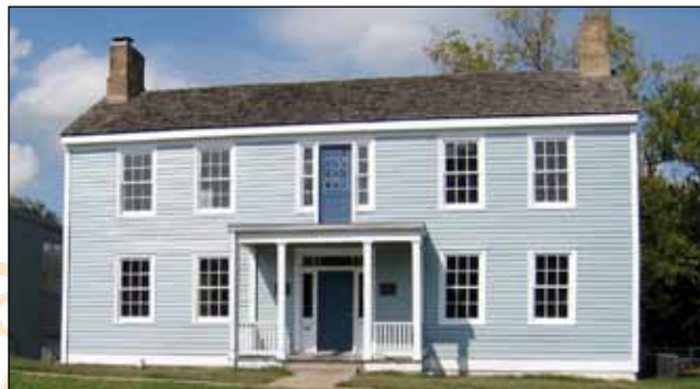
Fairfax House built circa 1841 in Rock Hill, Mo. by James Collier Marshall and Elizabeth Kyle McCausland Marshall.
