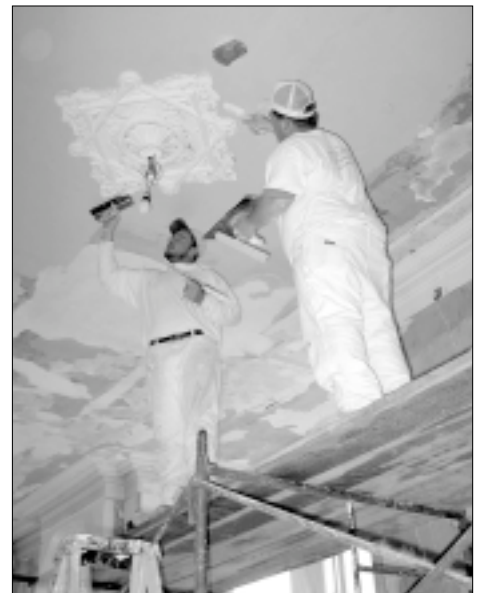
In January, plasterers began working on the Parlor ceiling.
