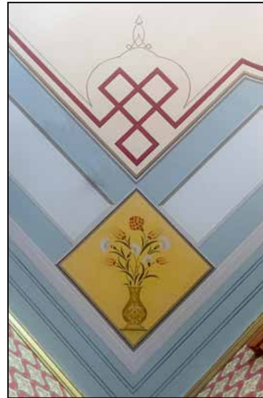
Dining room corner detail AFTER
