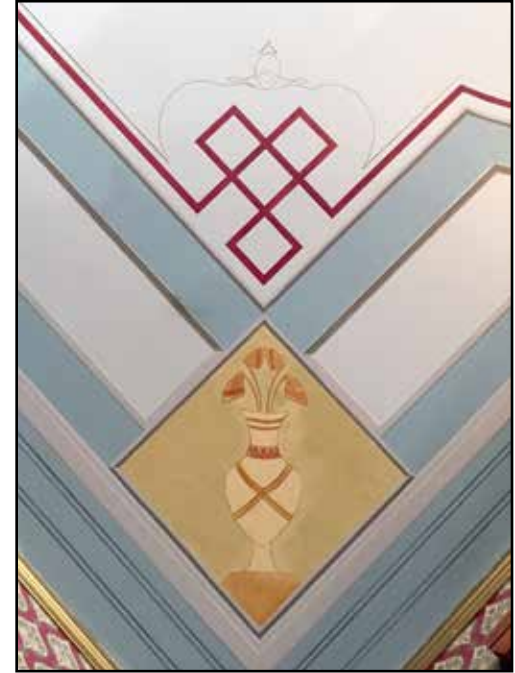
Dining room corner detail BEFORE
