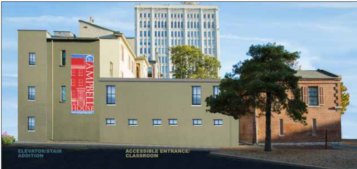
Photo rendering of the back of Campbell House showing the expansion to the Museum—the tall elevator and stair addition (at left) and accessible entrance lobby and classroom (center).
