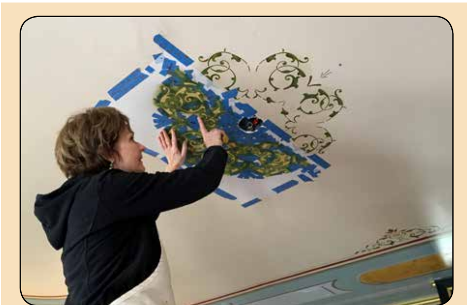
Artist Cindy Lugg stencils the ceiling medallion. (above) The completed medallion before the installation of the light fixture. (top)
