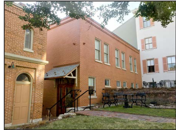
(top) The east wing of the completed expansion houses an accessible entrance, new Museum Store, a small lobby and multipurpose classroom.
